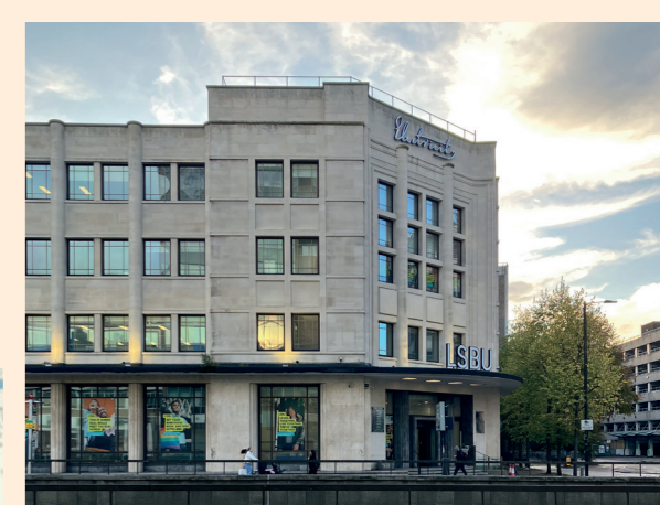
Electricity Showrooms and Offices (c. Allies and Morrison)
