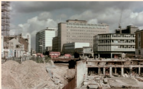
Redevelopment underway in Croydon, c.1960s (Source: BFI)
