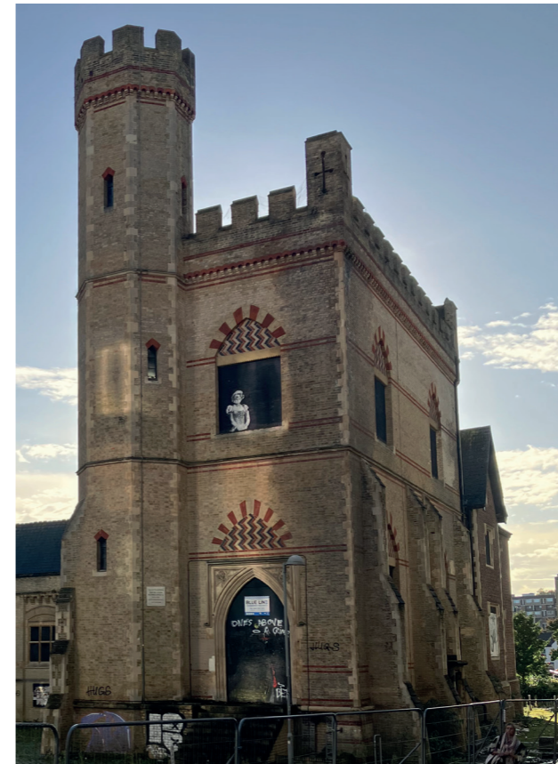
The Surrey Street Pumping Station
