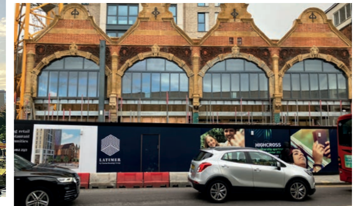
Station Road mixed use re-development
